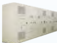
Control room and power distribution system
