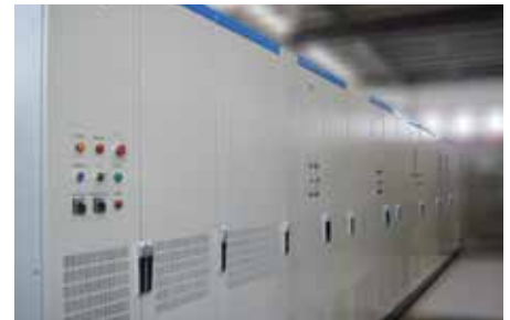
• Low voltage inverter (re-generation)
