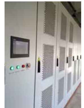
• MVD1000 for circulation water pump
