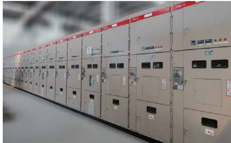
• High Voltage Distribution Cabinet
