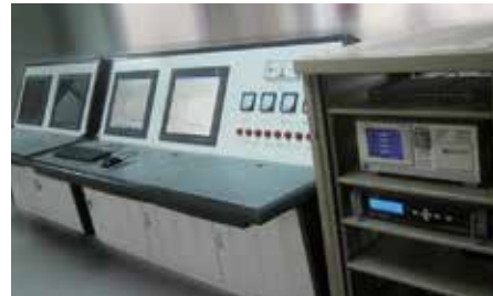
• Central control room
