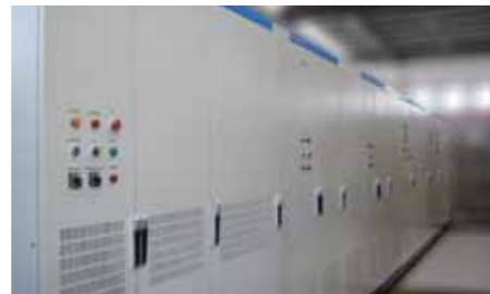
• Inverter to accompany in test
