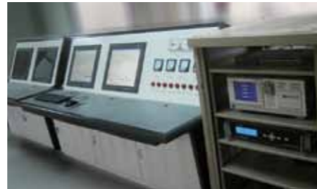
• Central control room
